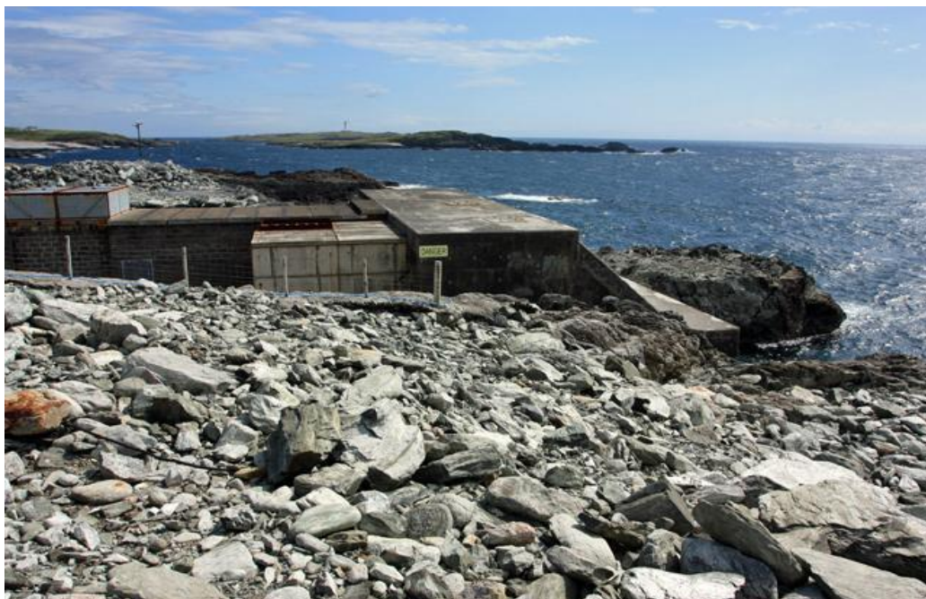
Fig. 7.10 Vista da central LIMPET (by Peter Church / CC-BY-SA-2.0, via Wikimedia Commons)
